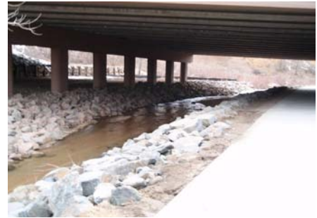
Figure 5-1 – CDOT Riprap along Plum Creek under the I-25 Bridge
