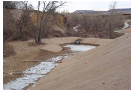
Figure 5-2 – CDOT detention pond that drains into Plum Creek assisted to keep approximately 36 tons of sediment out of Plum Creek
