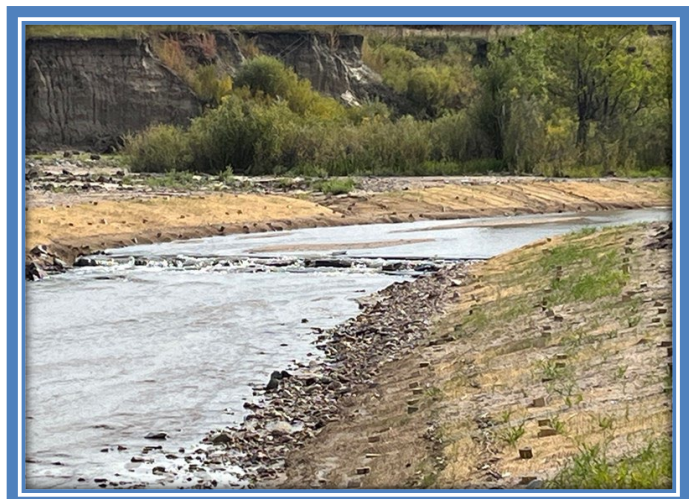
Figure 31. Drop 3 Completion with Grass Growing.
