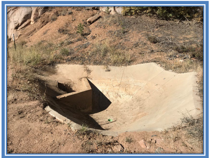
Figure 28. Sediment Trap after cleanout.
