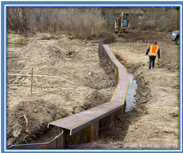
Figure 30. Installation of Sheet Pile and Cap Drop 3.
