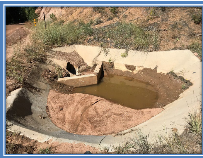
Figure 27. Sediment Trap before cleanout.
