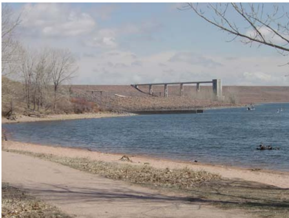
Chatfield Reservoir With Outlet Structure
