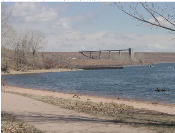
Chatfield Reservoir With Outlet Structure
