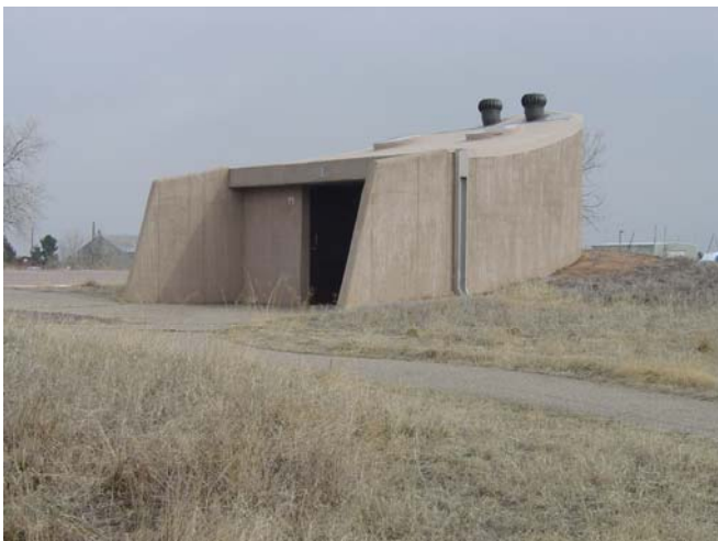
Suspected illicit wastewater source at Chatfield State Park
