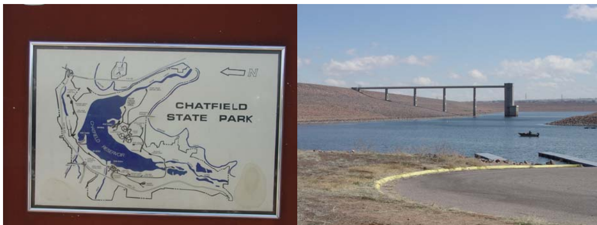
Figure 8 Outlet Structure at Chatfield Reservoir
