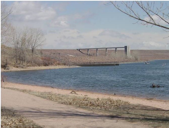
Chatfield Reservoir With Outlet Structure
