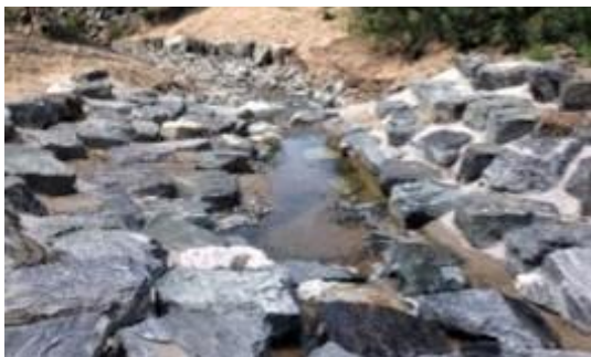
After: Control structures with riprap lining.
