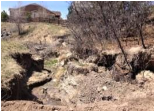
Before: Stormwater runoff channel.
