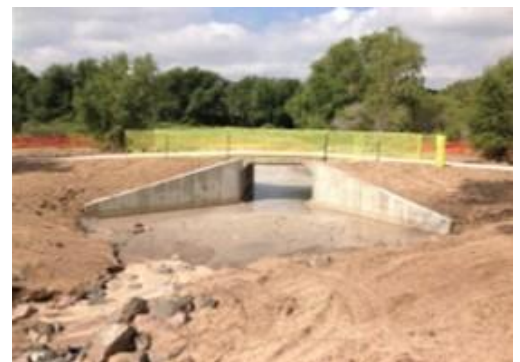
After: 10'x6' Box culvert at the East Plum Creek Trail.
