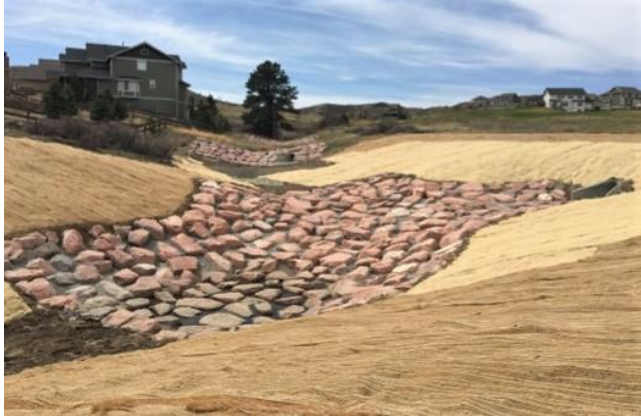
Grouted boulder drop structure.
