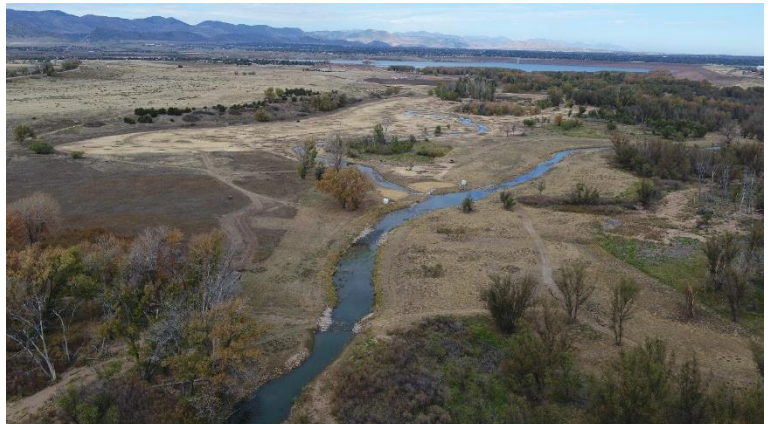
Downstream view of completed environmental mitigation work on Plum Creek looking toward Chatfield Reservoir.
