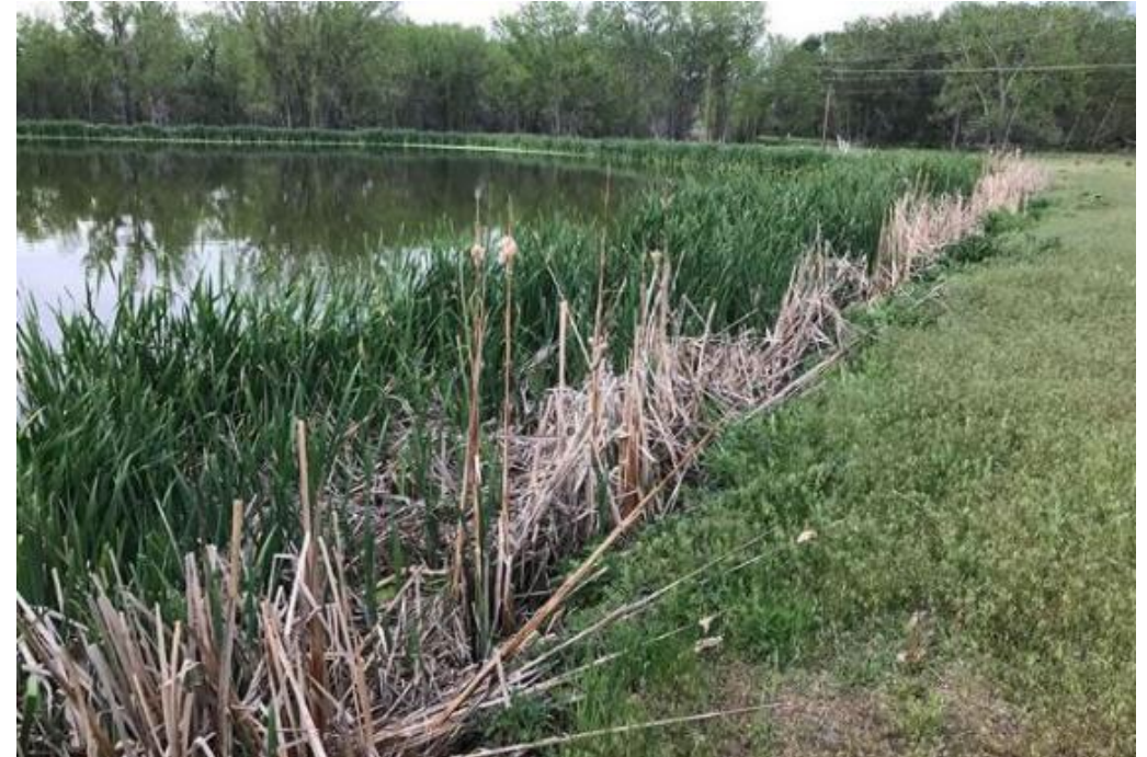
Louviers Wastewater Treatment Lagoon
