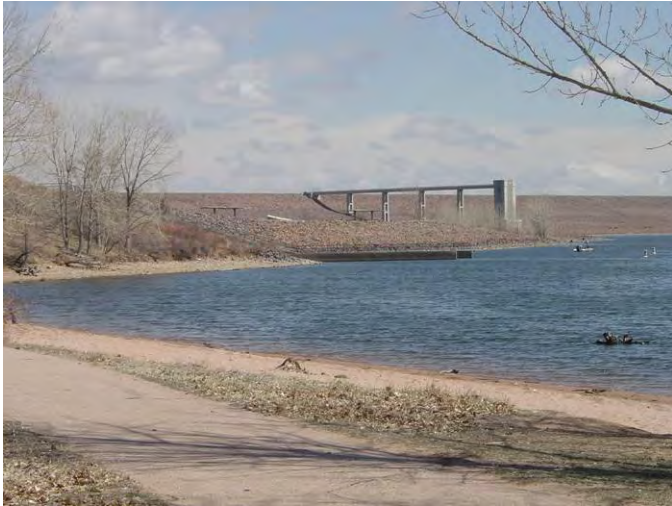
Chatfield Reservoir With Outlet Structure
